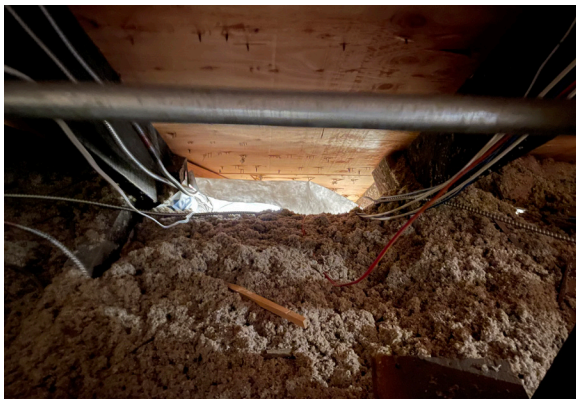
Figure 1-340. Loose insulation at perimeter of Attic I 300. Light is visible from Storage 205B below. (EAV, 08/24/2021)
