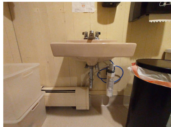
Figure 1-388. Second Level Lavatory Filter (JSW 8/24/2021)
