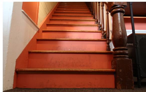
Figure 1-284. Facing north at the bottom of the stairs to the second floor. Note missing trim at replaced risers. (EAV, 08/24/2021)
