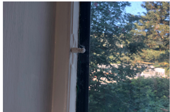
Figure 1-63. Windows are painted shut. (BM, 08/24/2021)
