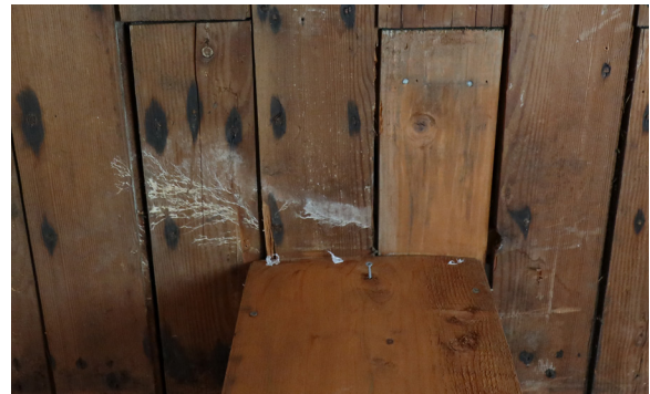
Figure 1-286. Growth on ceiling boards near the plumbing chase in Museum I 102. (EAV, 08/24/2021)
