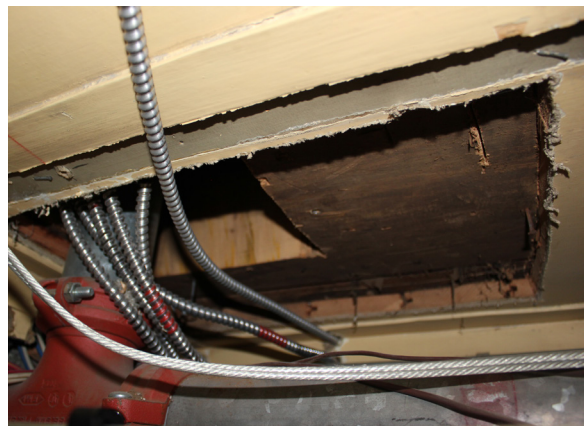
Figure 1-352. Second floor beam of the Magazin on the east half of the structure. Note the large hole cut in the beam to allow the piping to pass up to the second floor (CBB, 08/26/2021)
