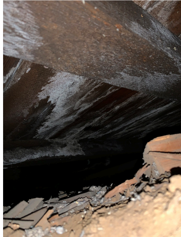
Figure 1-353. Second floor framing cavity of the Magazin on the east half of the structure. Note the 4x4 joists at the top of the cavity and the mold or water staining visible on the wood members (CBB, 08/25/2021)
