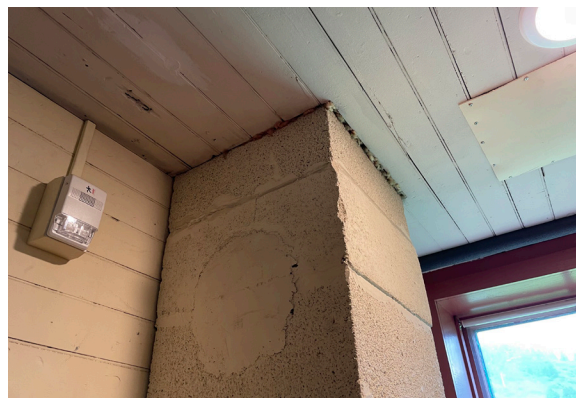
Figure 1-328. Patched ceiling and abandoned chimney in Stair Hall 200. (KAC, 08/24/2021)
