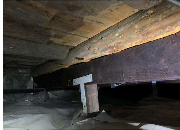
Figure 1-349. First floor framing of the Magazin west of the interior log wall. Note the deck boards framing to a dropped log beam that is now supported by a continuous dropped creosote treated member (CBB, 08/25/2021)
