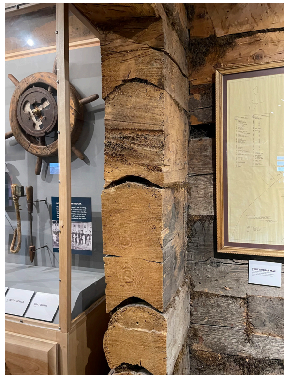
Figure 1-215. Hewn logs and moss chinking at CO 103. (KAC, 08/24/2021)
