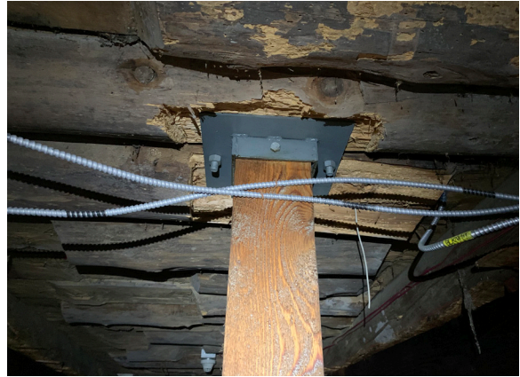
Figure 1-351. Timber post supporting dropped second floor glulam beam added in the 1980s as seen from the crawlspace (CBB, 08/24/2021)
