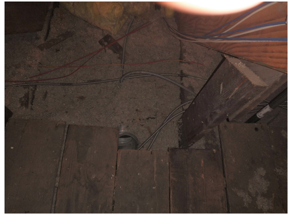
Figure 1-381. Second Level Restroom Exhaust Into Attic (JSW 8/24/2021)
