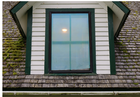
Figure 1-163. Deteriorated sill at Window 30, Type C. (EAV, 08/24/2021)
