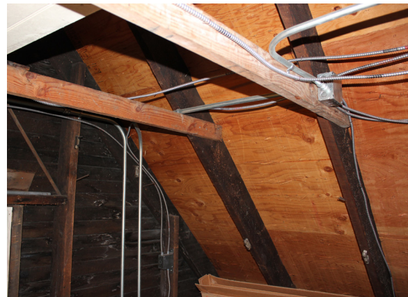
Figure 1-362. Roof framing of the Magazin. Note the rafters, collar ties, and plywood sheathing (CBB, 08/26/2021)
