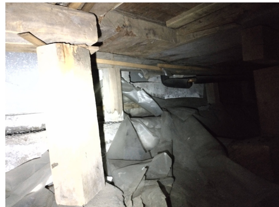
Figure 1-387. Damaged Cast-Iron Waste Pipe (JSW 8/24/2021)
