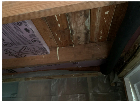
Figure 1-347. Interior face of the south wood stud foundation wall of the Sun Porch as seen through the plastic sheeting (CBB, 08/24/2021)
