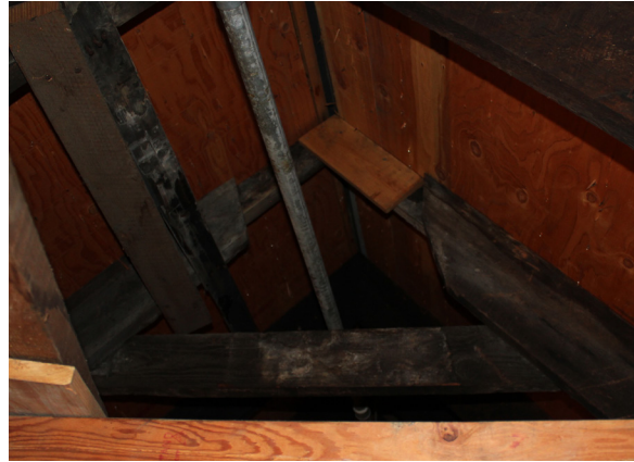
Figure 1-367. In one location, the rafters have been cutback from the peak of the roof and sistered (CBB, 08/26/2021)
