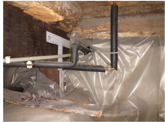
Figure 1-376. Hydronic Piping In The Crawlspace (JSW 8/24/2021)
