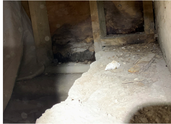
Figure 1-346. Interior face of the north wood stud foundation wall of the Alcove. Note the water staining and deterioration at the base of the wall (CBB, 08/25/2021)
