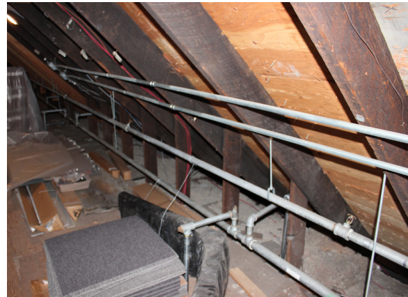
Figure 1-364. Verticals hanging the attic floor joists from the rafters (as seen behind the piping). (CBB, 08/26/2021)
