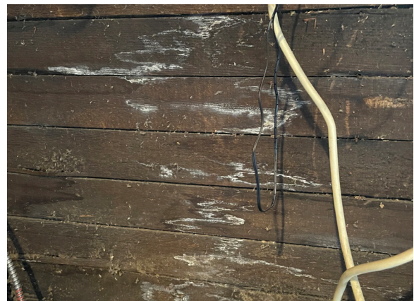
Figure 1-343. Smoke stain and efflorescence on exposed sheathing at the east wall of Attic I 300. (EAV, 08/24/2021)
