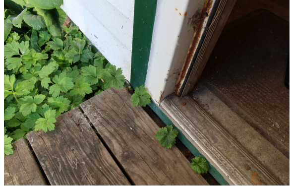
Figure 1-207. Rust at frame of Door 110. (EAV, 08/24/2021)
