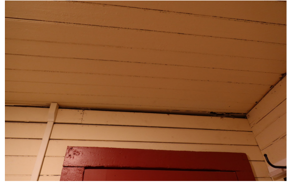
Figure 1-335. Gap at the top of the south wall of Staff Restroom 207. (EAV, 08/24/2021)
