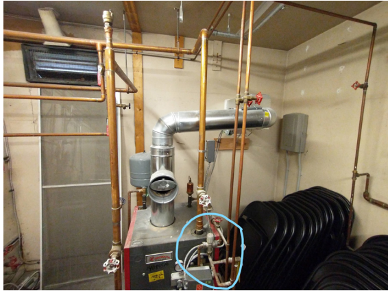
Figure 1-389. Domestic Hot Water Mixing Valve (JSW 8/24/2021)
