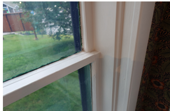
Figure 1-193. Window 15, interior. Note visible paint on glazing and sashes painted shut. (EAV, 08/24/2021)
