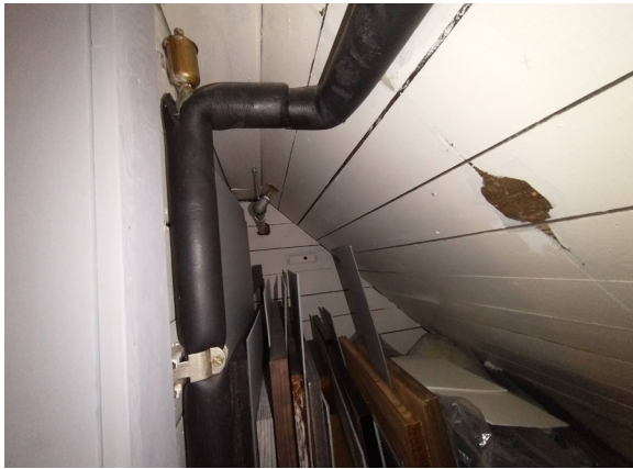
Figure 1-378. Hydronic Piping on The Second Level (JSW 8/24/2021)
