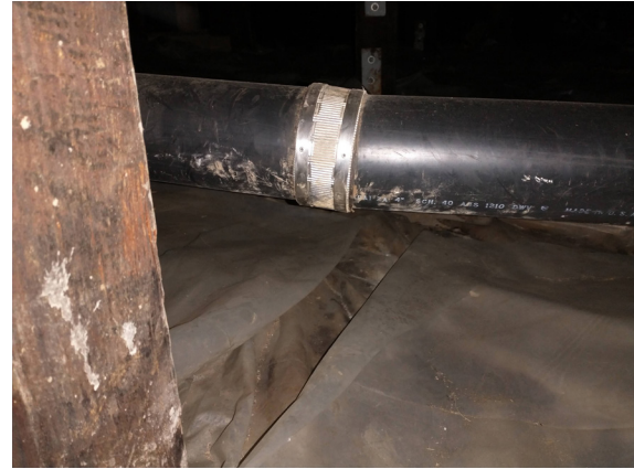
Figure 1-386. ABS Piping in Crawlspace (JSW 8/24/2021)
