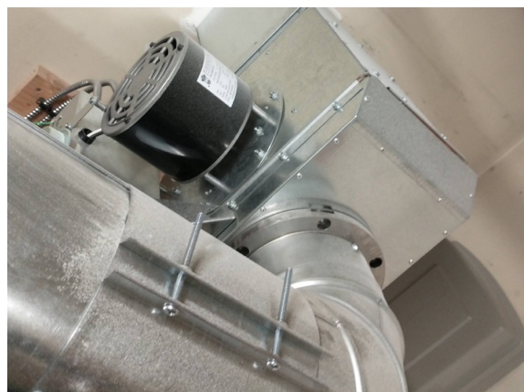
Figure 1-372. Boiler Flue Draft Inducer (JSW 8/24/2021)
