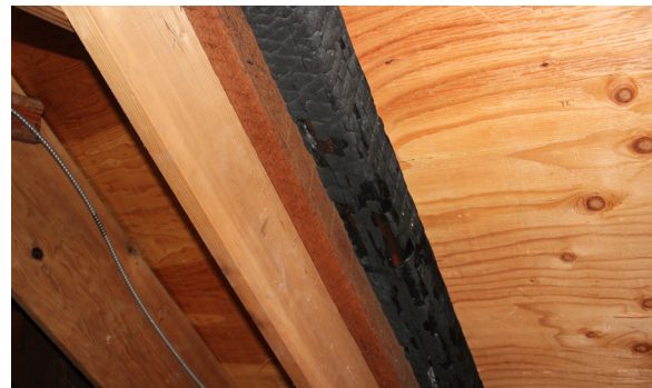
Figure 1-363. Charred 4x4 rafter with sisters (CBB, 08/26/2021)
