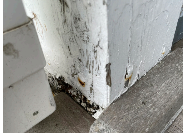
Figure 1-150. Deteriorated column base. (KAC, 08/24/2021)
