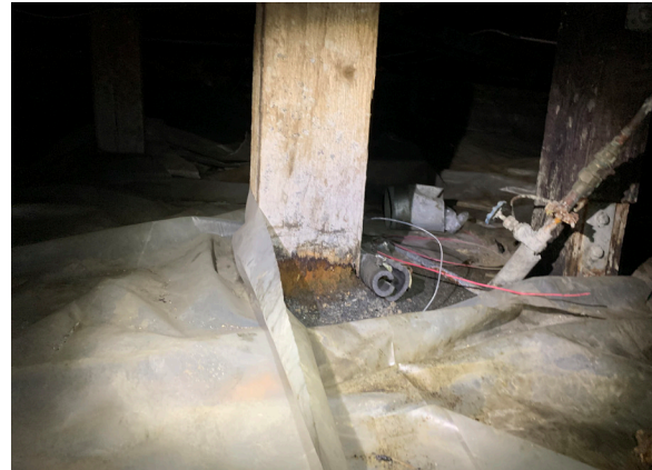
Figure 1-355. Deteriorating base of a post supporting the first floor of the Magazin (CBB, 08/25/2021)
