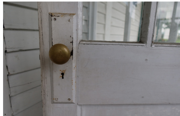
Figure 1-206. Missing and worn paint on and near hardware of Door 103B, exterior. (EAV, 08/24/2021)
