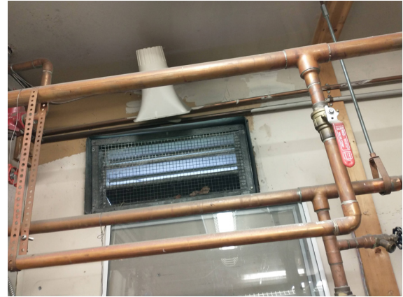
Figure 1-374. Combustion Air Louver (JSW 8/24/2021)
