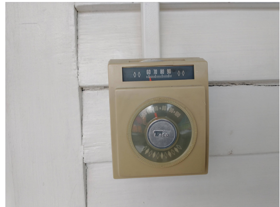
Figure 1-375. Hydronic Thermostat (JSW 8/24/2021)
