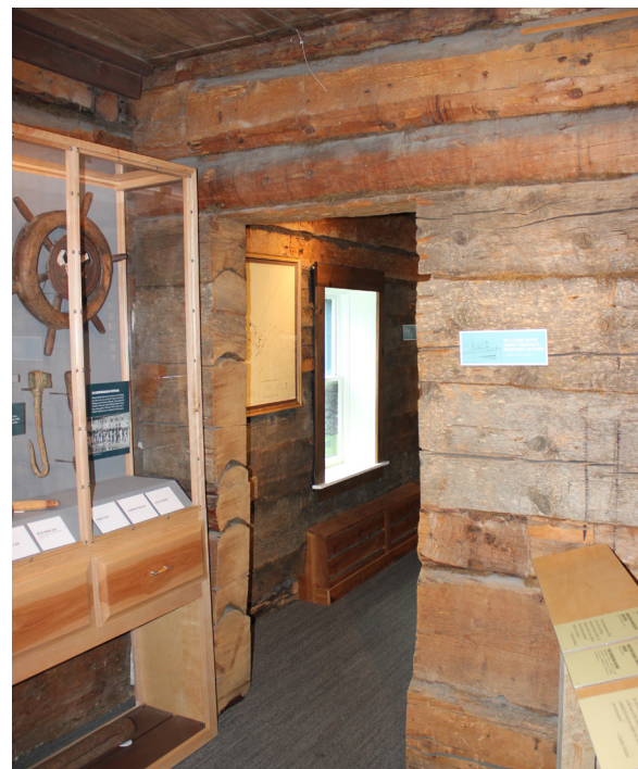
Figure 1-369. Opening created in the interior log wall after the original construction (CBB, 08/25/2021)
