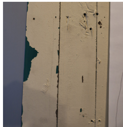
Figure 1-336. Thickly applied and missing paint at wall boards in Director's Office 208. (EAV, 08/24/2021)
