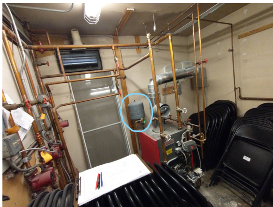
Figure 1-373. Poorly Supported Expansion Tank (JSW 8/24/2021)
