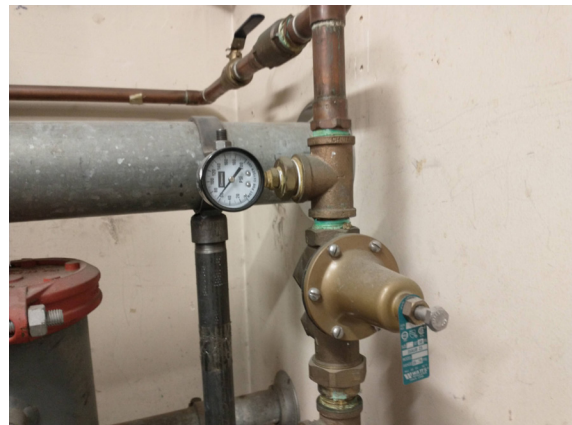
Figure 1-384. Domestic Water PRV (JSW 8/24/2021)
