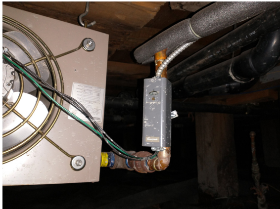
Figure 1-379. Unit Heater in Crawlspace (JSW 8/24/2021)
