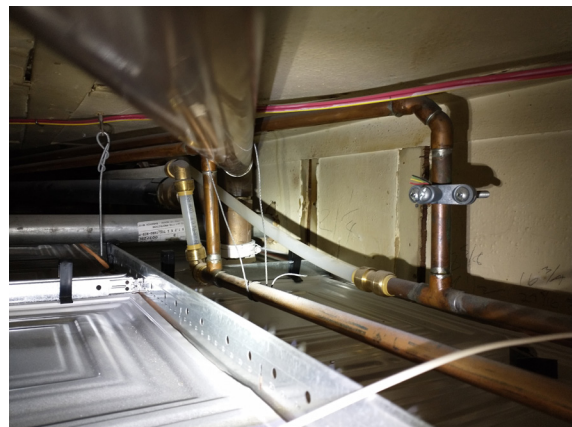
Figure 1-385. Copper to PEX Domestic Water Transition (JSW 8/24/2021)
