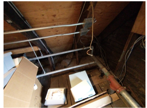
Figure 1-401. Attic Fire Sprinkler Heads and Piping (JSW 8/24/2021)
