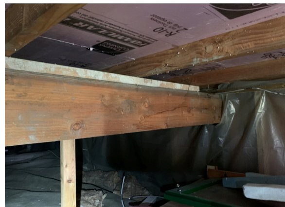
Figure 1-354. Joists and dropped beams of the first floor of the Sun Porch (CBB, 08/24/2021)
